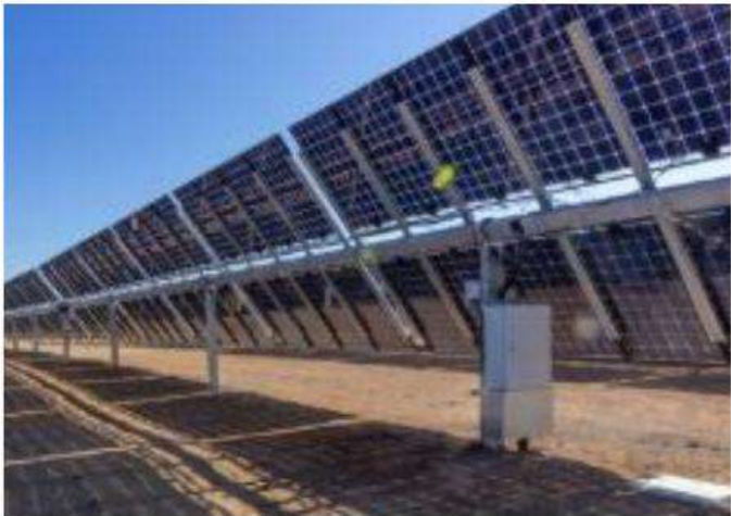
The total area of the plots is 26.9 hectares. Direct connection to the plant's distribution network is being considered.
